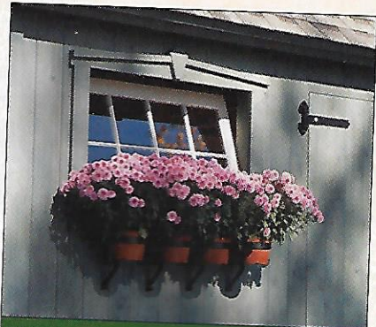
Barn-sash windows pivot at the sides to allow for ventilation. Siding, doors and trim are made of cedar.
