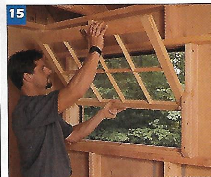
15 Slip the barn-sash window into the window frame and set it down on the sill. A simple barrel bolt holds it closed.
