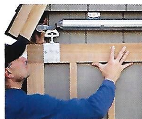
Door Installation p. 209
