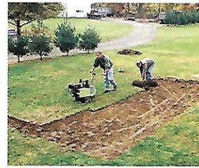
Site Prep and Footings p. 188
