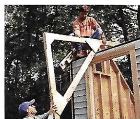
Roof Framing p. 138
