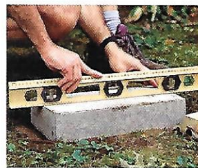
Solid-Block Foundation p. 126
